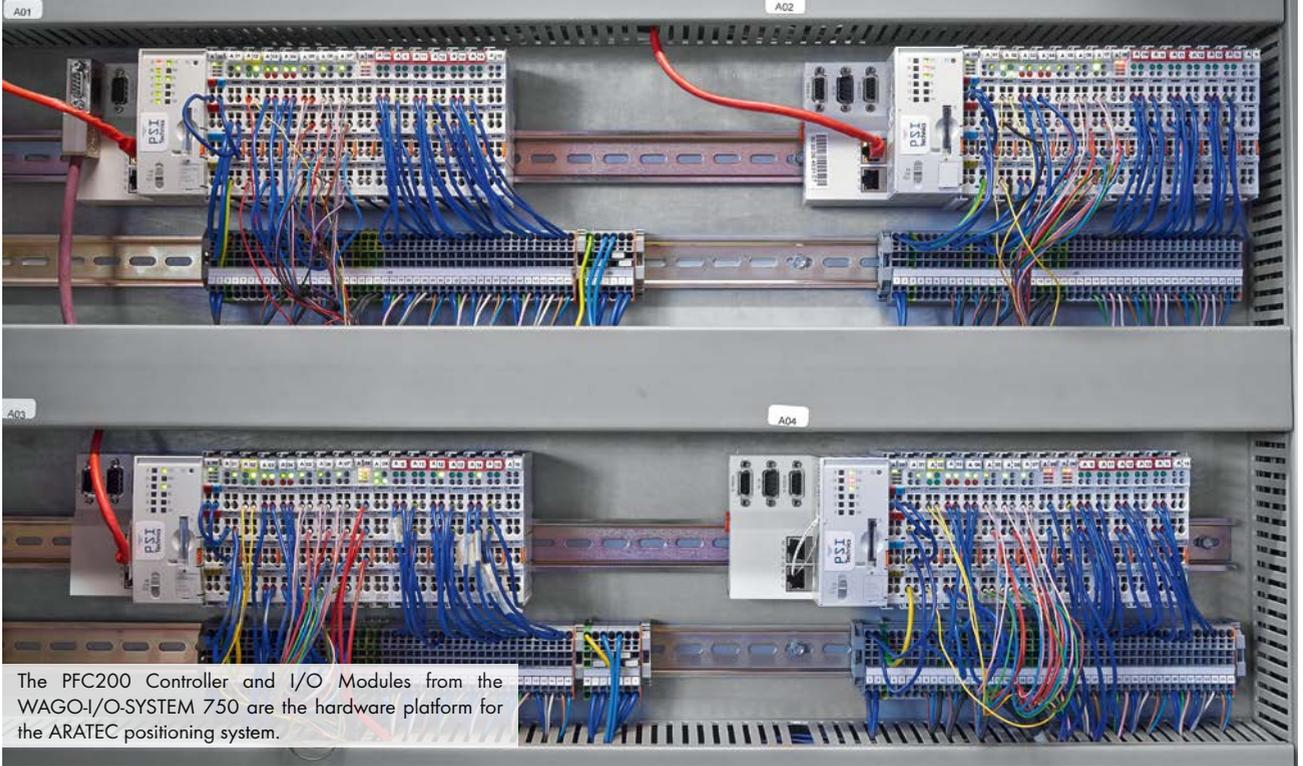
The PFC200 Controller and I/O Modules from the WAGO-I/O-SYSTEM 750 are the hardware platform for the ARATEC positioning system.
